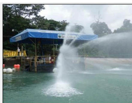
Powerful water jetting disintegrates sediments
